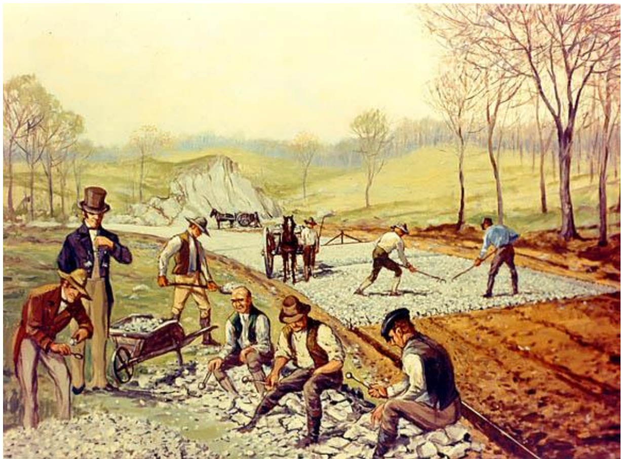
Building roads on the McAdam principle
